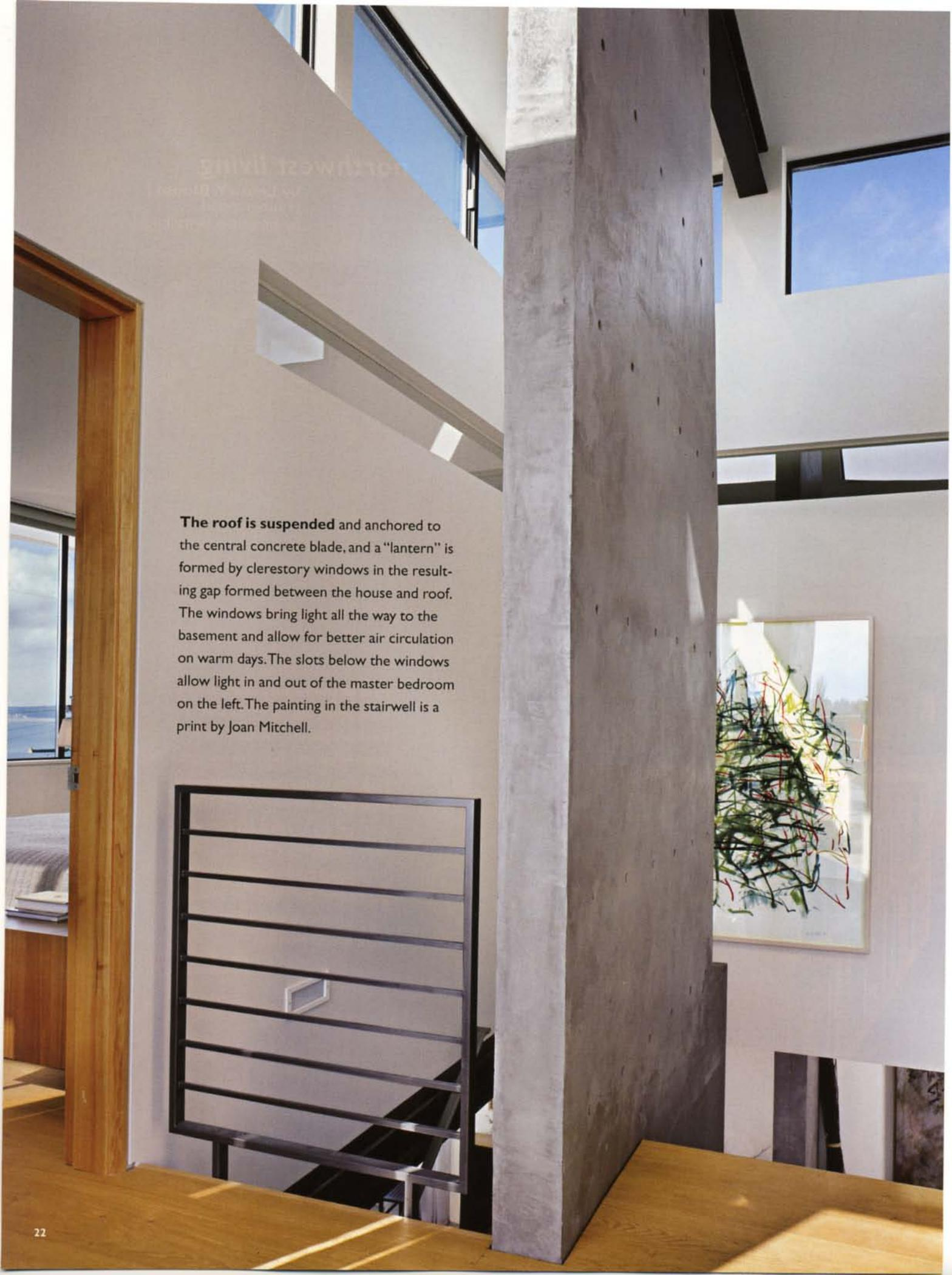
**The roof is suspended** and anchored to the central concrete blade, and a “lantern” is formed by clerestory windows in the resulting gap formed between the house and roof. The windows bring light all the way to the basement and allow for better air circulation on warm days. The slots below the windows allow light in and out of the master bedroom on the left. The painting in the stairwell is a print by Joan Mitchell.
